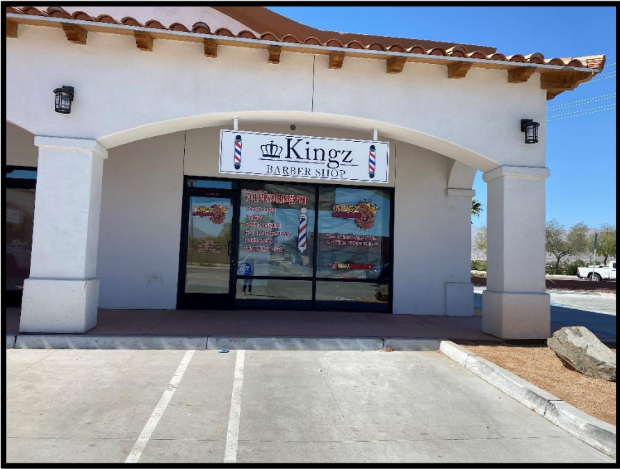
Close-up of hanging sign (metal frame box with wood sign face)
